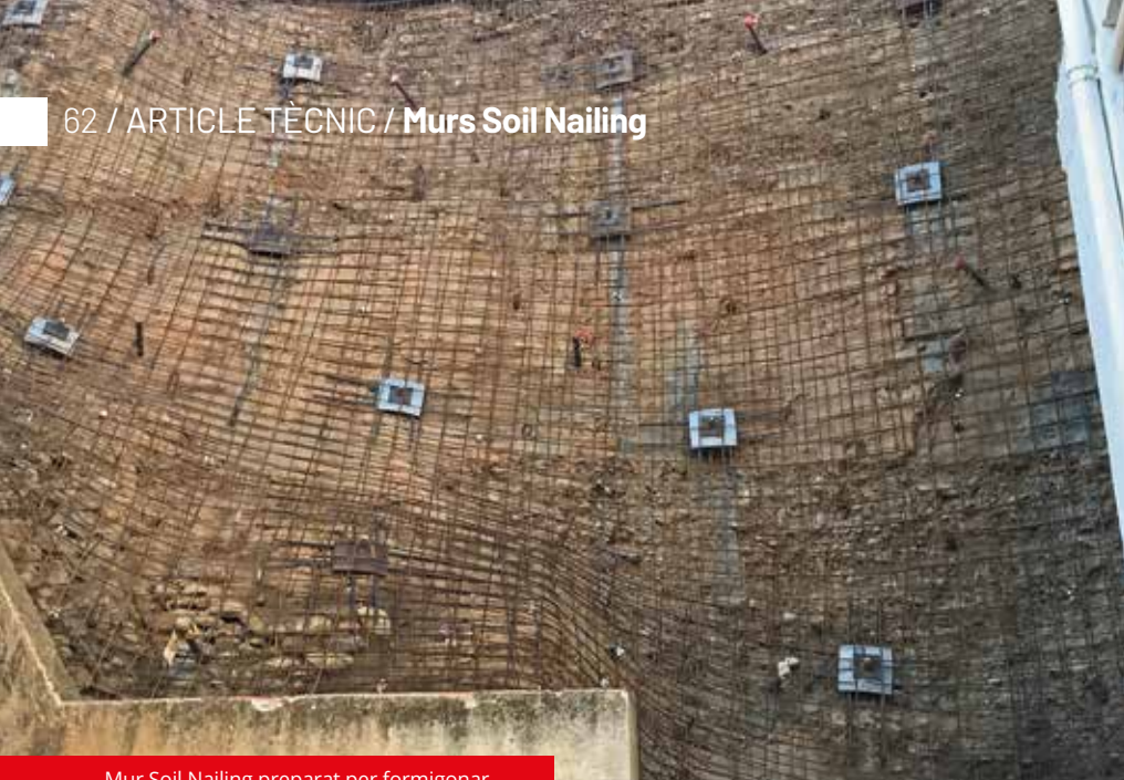
Mur Soil Nailing preparat per formigonar
